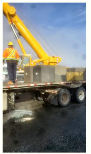
The first of 5 truckloads arrived at D Jetty. We are getting 110 of these – at 4600 lbs each that is 253 imperial tons. With what QHM is giving us in addition, that should round up over 300 tons anchoring the docks. The engineers say this should be enough for ground tackle! Thank you to Bethany, Ginette, Mike, Kurtis & Kevin for being onsite to meet the delivery trucks.
